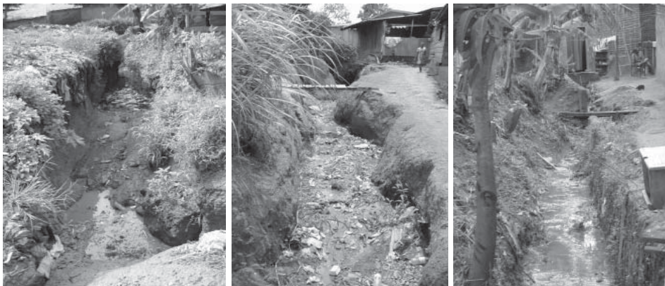
Side ground ditches dug by water during their flow, and of... ground drains worked out by the inhabitants. ©Nguendo Yongsi, 2006
