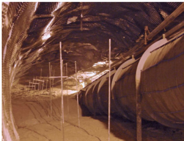
Figure 3.12. Decay pipe. Image taken from [6].
