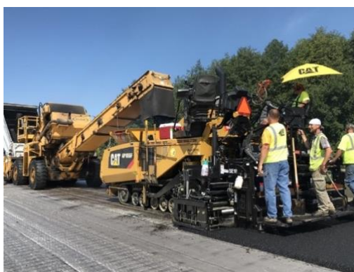
Figura 1: Elaboración de carpeta asfáltica. "US 2 Paving: Asphalt paver on Hewitt Avenue Trestle" by WSDOT is licensed under CC BY-NC-ND 2.0.
